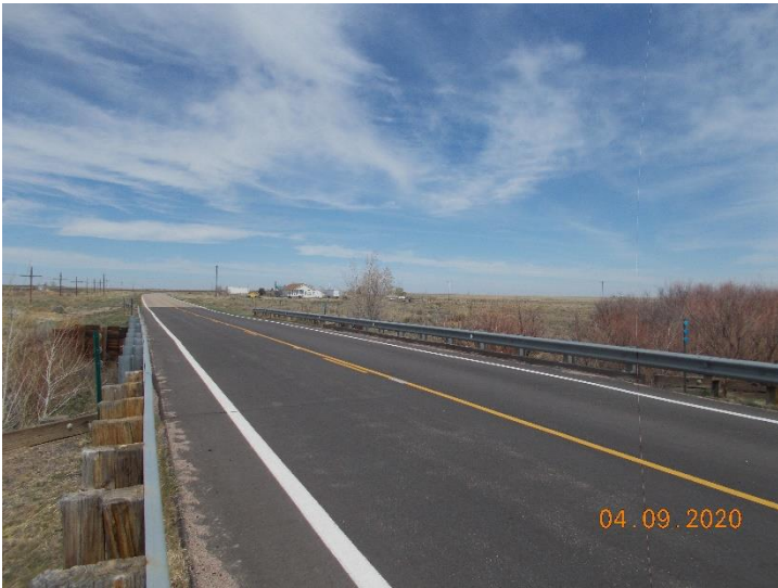
View of bridge O-19-D looking north.
