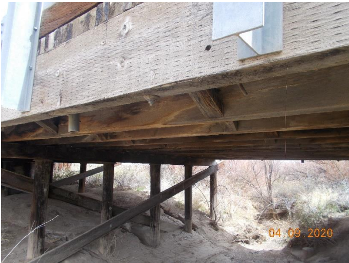
View beneath bridge O-19-D.
